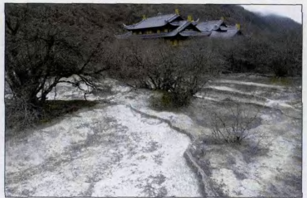
照片 11 五彩池景区下游干枯变黑的钙华池 Photo 11 Dried and blacked travertine rimstone pools at Wucaichi
